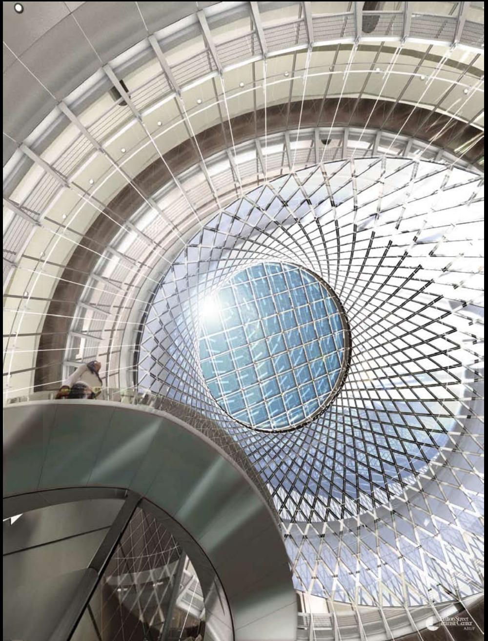
Image courtesy of NYCT CC/Arup
