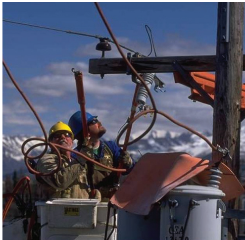
Overhead maintenance. Image courtesy of Municipal Light & Power.
