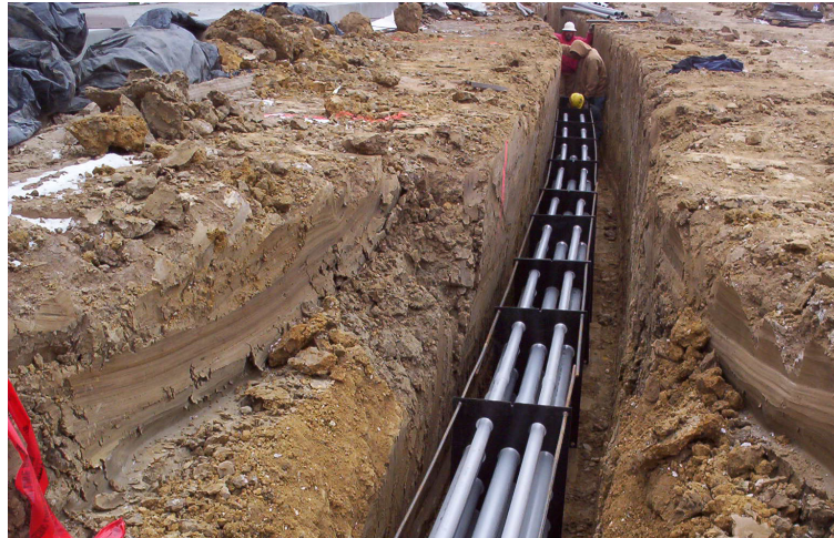
Construction of ducts. Image courtesy of Kansas City Board of Public Utilities.
